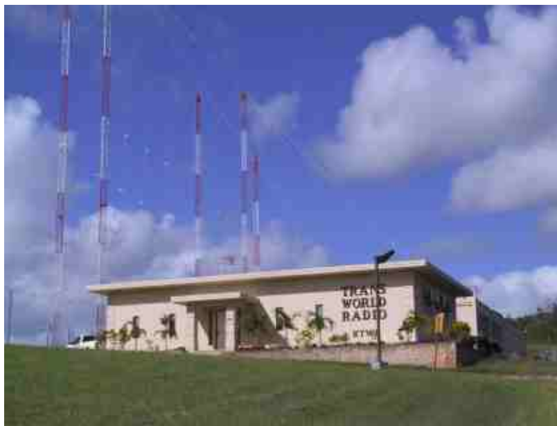
KTWR office building and part of the antenna field
